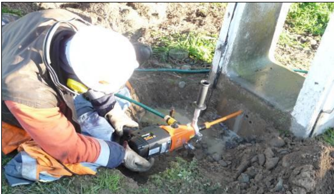
Figure 5: Diamond drilling a Vierendeel pole.
