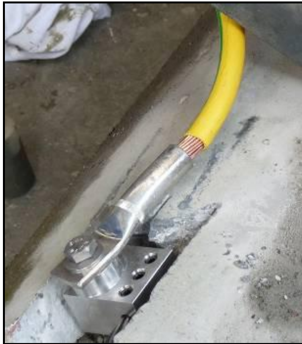
Figure 10: Hollow Spun Pole top bonding connector (Prior to mortaring into pole wall).
