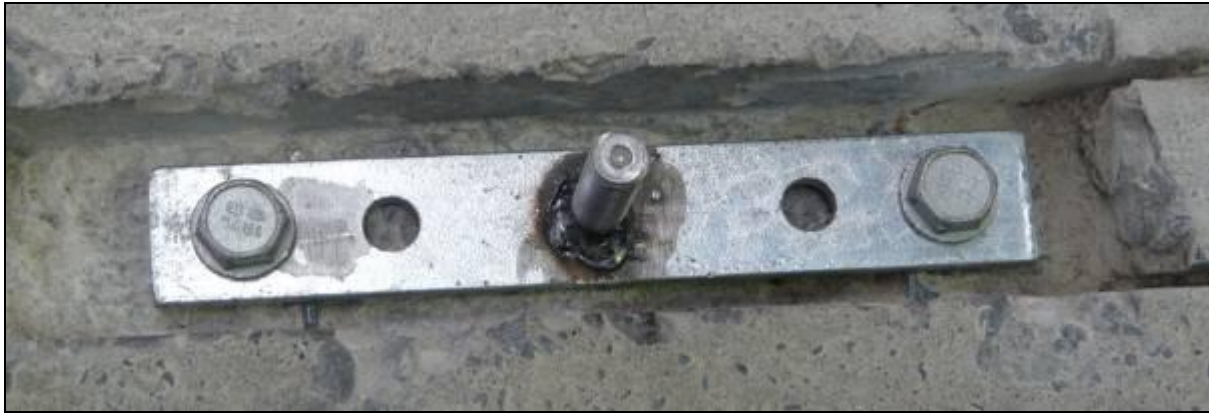
Figure 8: Design 1A Bonding Bracket for Hollow Spun Poles.
