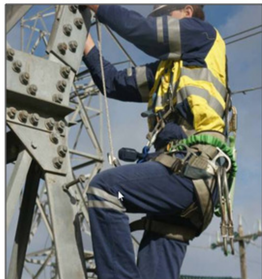
Photos show workers climbing using wire type attachment systems.
